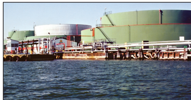
Castle Oil Corp., Deep Water Terminal, Bronx, N.Y.
