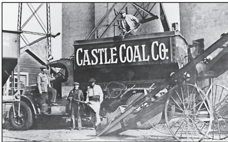
Original Coal Silo, Bronx, N.Y. Castle Oil Corp. in the 1930s
